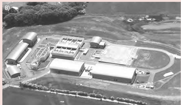
Figure 12.21 (A) Hydrated aluminum sulfate as seen using polarized light. (B) A modern water purification plant. Courtesy of United Utilities, Warrington, UK.
